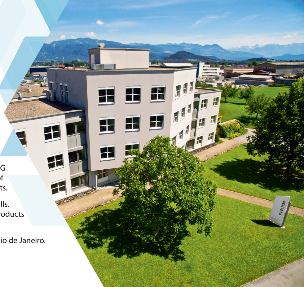
COLTENE Headquarter, Altstätten / Switzerland
